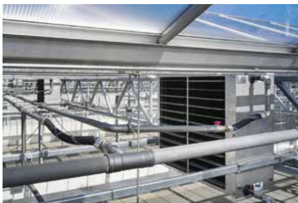
The incredible strength of the steel pipes and the Megapress connection pieces means piping can be installed below the hall ceilings with a minimal number of fixed points.
