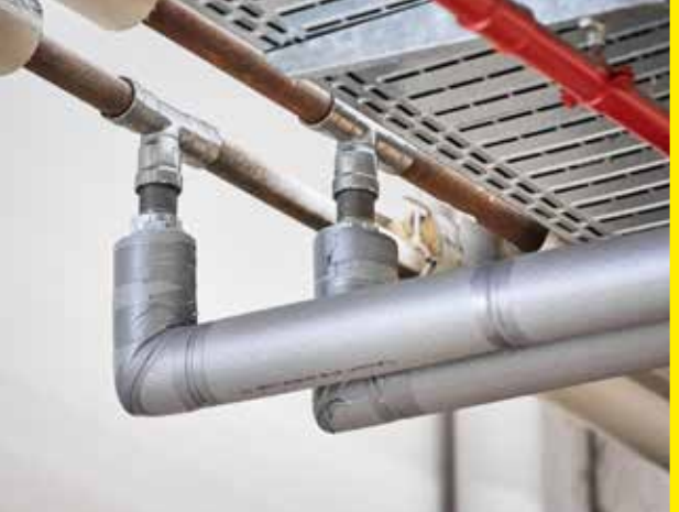
Pressed in seconds rather than laboriously welded: Megapress outlets in the production hall.
